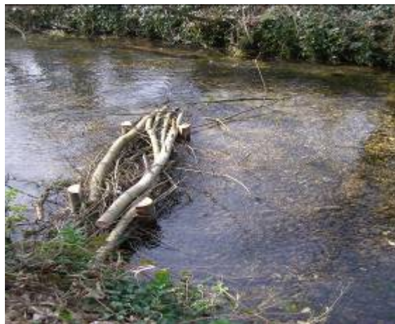
One of the woody debris structures installed
