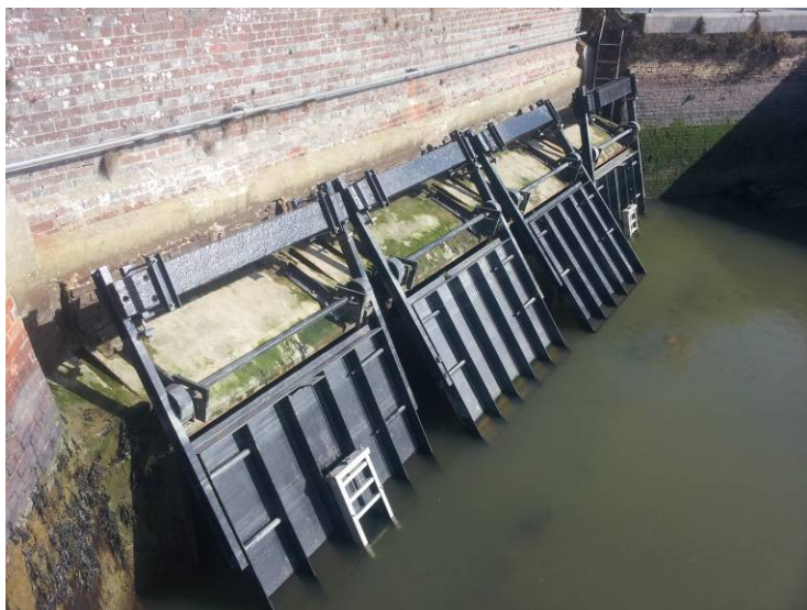
River Meon tidal gates improved for fish passage and wildlife
