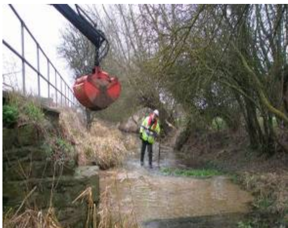
New gravels going into the River Churn
