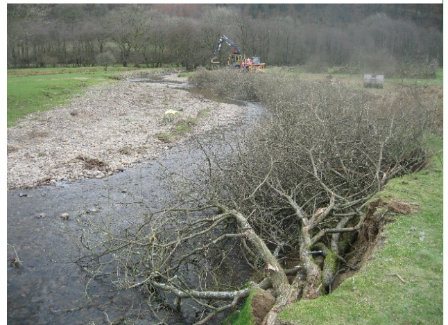
Figure 1: Large scale brash installation (Wye & Usk Foundation) responsible for increases in juvenile
